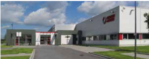
Ultra-modern production site in Gladbeck
